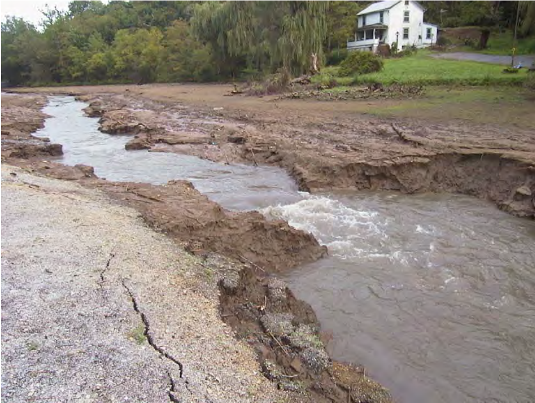
Photo 5: Nickpoint showing continuing upstream erosion above Reedsville Milling Company Dam.
